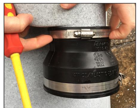
14. You will need to loosen the jubilee clip on the 3" side and slide this up to ensure a tight fit.
