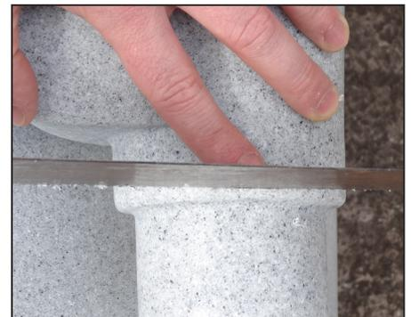
11. Using a hacksaw, cut across the inlet at the measurement shown.
