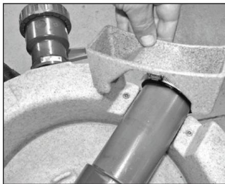
5. Remove the 90mm return pipe assembly from the EazyPod body.
