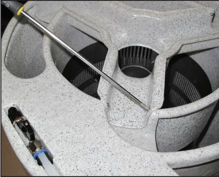
1. Remove the overflow assembly and safely store the 3 screws which secure it
